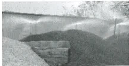
Sprinkling Aggregate in a Stockpile
